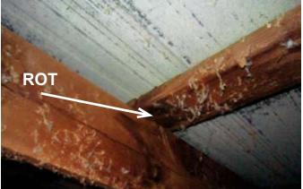
Moisture is the enemy in a poultry house attic. Humid "bird air" like that leaking around the attic access panel in the left photo causes the metal nailing plates to corrode and wooden members to show early signs of rot. Roof leaks seen in the right hand photo can also cause truss members and purlins to rot.
