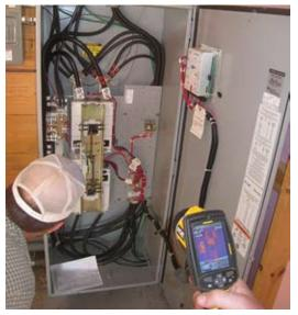
Automatic Transfer Switch – The brain of the transfer switch is probably the electronic component on the modern poultry farm most frequently damaged by lightning or by power surges.
