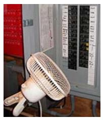
to heat up. An infrared temperature gun is a relatively inexpensive and guick way to spot overheating breakers or other gear. (See "Tools of the Trade" at www.poultryhouse.com.) If breakers are hot or are tripping often, we need a qualified electrician to tell us why they are hot and how to fix the problem.
