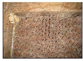
Insects, dust, dirt, and dander can quickly clog evaporative cooling pads during summer months. Keeping the pads clean greatly improves airflow and bird cooling.
