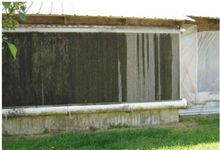
to burn out. Reliable recirculation pumping is so important some growers use two pumps on each system. Where there is only one pump, paying attention to maintenance is especially critical. Sump pump levels should also be checked and adjusted if needed to make sure enough water is available for good cooling.
