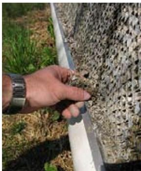
Grass clippings, leaves, dirt, and other materials must not be allowed to collect on pads. Buildup like this will stop up a filter in a matter of seconds if allowed to enter the system water storage.
