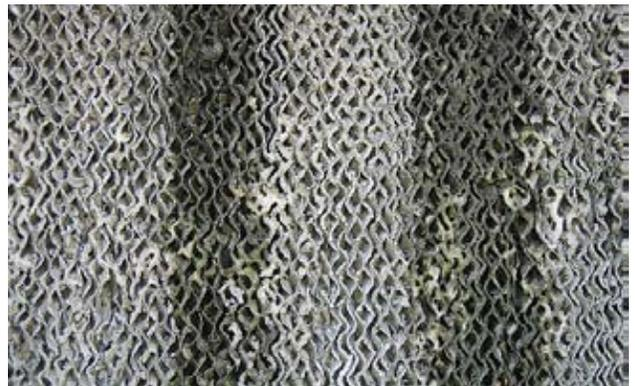
Clogged pads cause severely reduced cooling, increased electrical costs, and poor feed conversion and flock performance; not to mention decreased pad life if the problem is not corrected.
