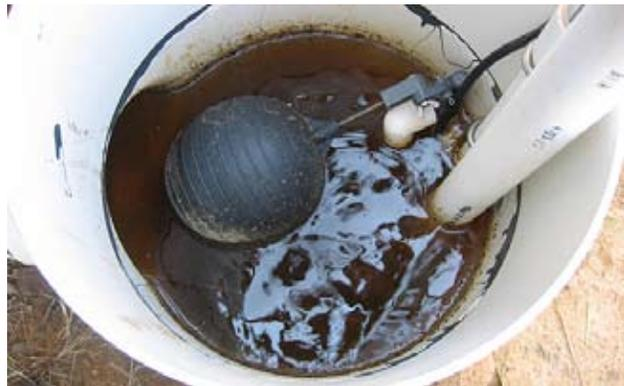
Dirty water leaves all its dirt on the pad as the water evaporates. This water needs to be dumped and the system cleaned out. Usually, system water should be dumped and replenished on a weekly basis.
