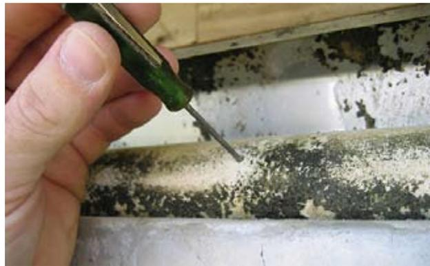
Clogged holes in distribution headers can often be cleared by poking a small screwdriver or other tool into the hole to remove the foreign matter.
