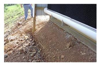
Failure to size house pads properly so they extend at least 5 feet from all sides of the house and projections such as evaporative cooling doghouses is a common serious problem in pad construction. This pad was not prepared properly, and should have been rejected by the grower and house contractor. Erosion is likely to cause (or has caused) serious damage here.
