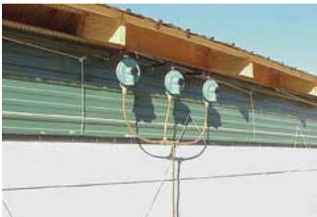
The trunk line from the gas tank and first stage regulator branches to serve three second stage regulators, which take gas at 10 psi and reduce the pressure to approximately 11-13 inches of water column. Second stage regulators should be located outside the house.
