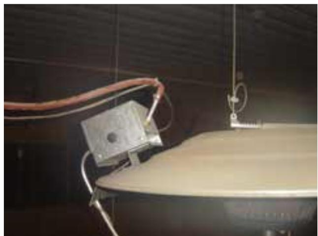
Photo above shows flexible gas hose to brooder pulled at a sharp angle so that it develops a kink, which will starve the brooder for gas, and also will be in danger of breaking at the kink point. Photo at left shows a spring-type anti-kinking device, which is good practice for all flexible hose.
