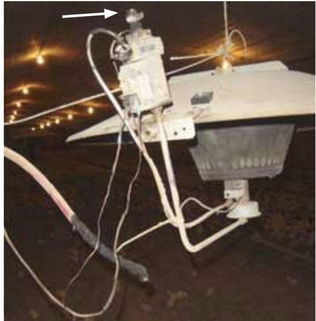
Above photo is a close-up of the picture on the front page, showing clearly the burnt end of the gas hose. Arrow shows where it was originally attached. Photo below shows gas hose running directly above the brooder, which risks fire if the hose comes in contact with the brooder when it is raised.
