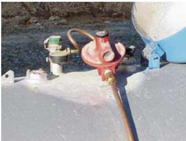
Photo at left shows a gas supply tank and the first stage regulator that steps the gas pressure down to approximately 10 psi for delivery to the poultry house through the trunk line.
