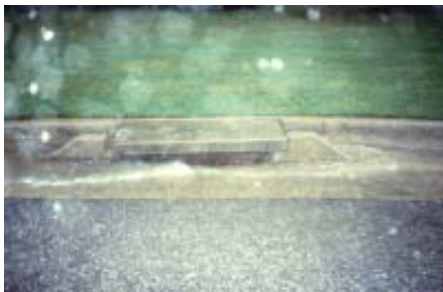
RUNOFF FROM STREETS AND LAWNS ENTERS STORM DRAINS AND FLOWS DIRECTLY TO STREAMS UNTREATED
