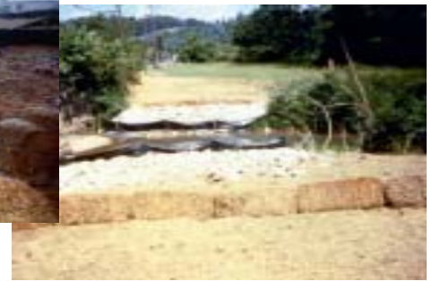
BMPs CAN DRAMATICALLY REDUCE EROSION AND STREAM SEDIMENTATION
