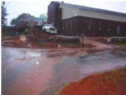
ERODED SOIL WASHING TO STORM DRAINS AND CREEKS.
