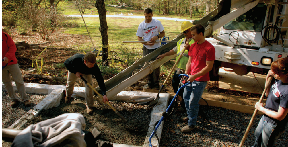
PERVIOUS POUR Students in building science classes installed pervious concrete pathways in the arboretum in 2011. Pervious concrete reduces stormwater runoff by capturing stormwater and allowing it to seep into the ground and is one of the Best Management Practices recommended by the EPA to manage stormwater runoff—a major issue in sustainable building practices.
