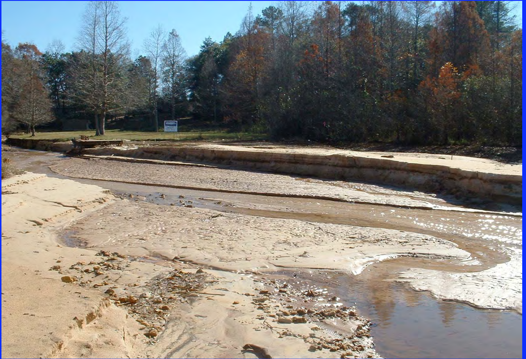
Sedimentation into Gantt Reservoir Covington Co. Alabama
